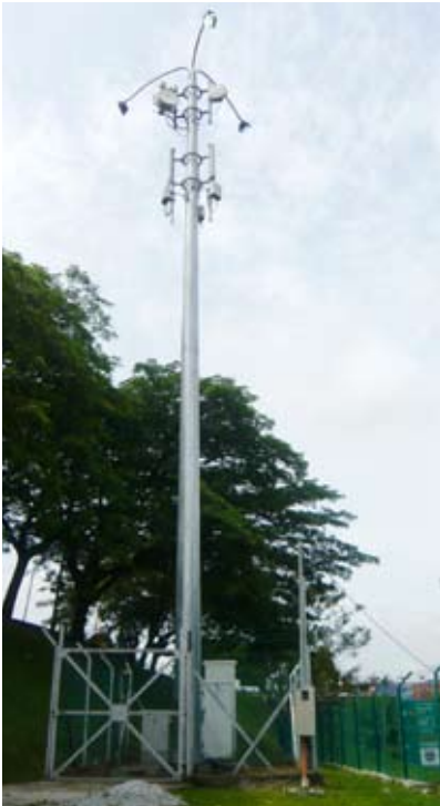
A type of telecommunication site for wireless services such as 3G and LTE
