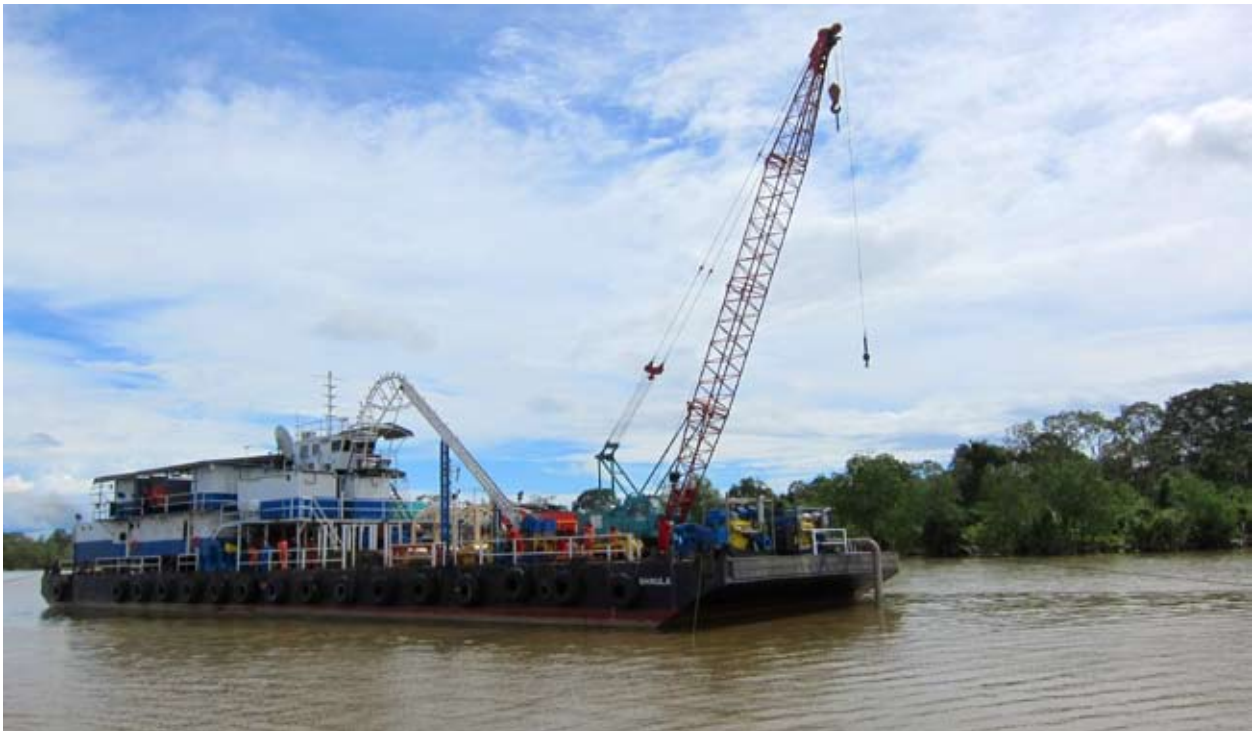
A special vessel used to lay the submarine cable
